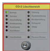
Display board and optional key switch for one extinguishing zone
